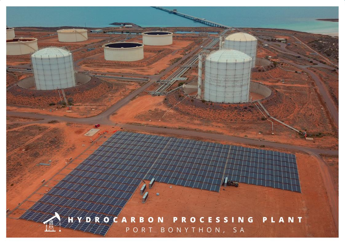
Port Bonython is home to a hydrocarbon processing facility, located 16 km outside of Whyalla, SA. Our client was looking for a cost effective, simple solution to provide over 2MWp of solar power to the site, in order to reduce their overall cost of energy. The rural nature of the site carried with it logistical and financial risks, as sending labour and equipment to site is expensive and time consuming exercise.
